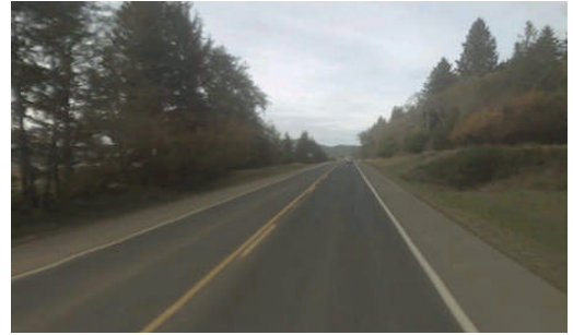
Photo 8 Route SW-1 SR-4, west of the town of Naselle.
