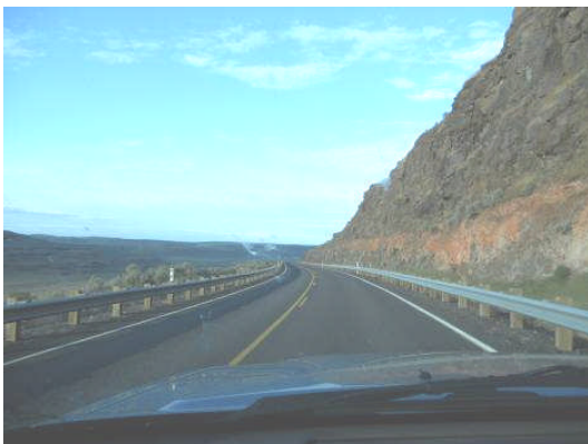
Photo 5 Looking east along SR-260, west of Kahlotus.
