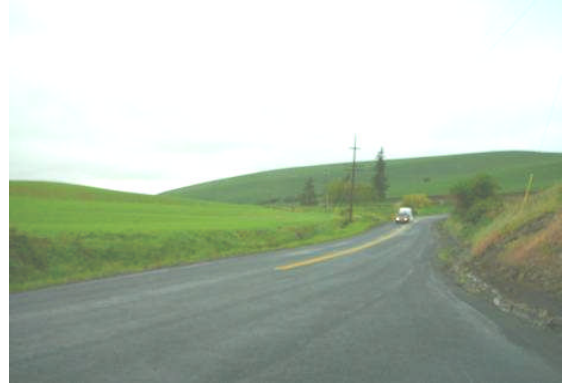
Photo 3 Route SE-2 Typical Terrain South of Waitsburg
