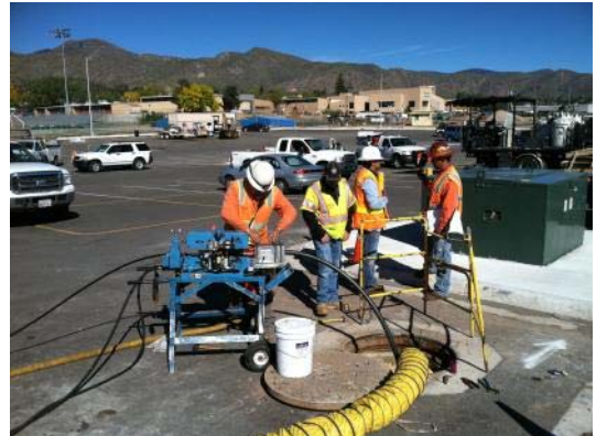
REDI Net crew members deploy new fiber as part of the more than 150-mile network project in north central New Mexico.
