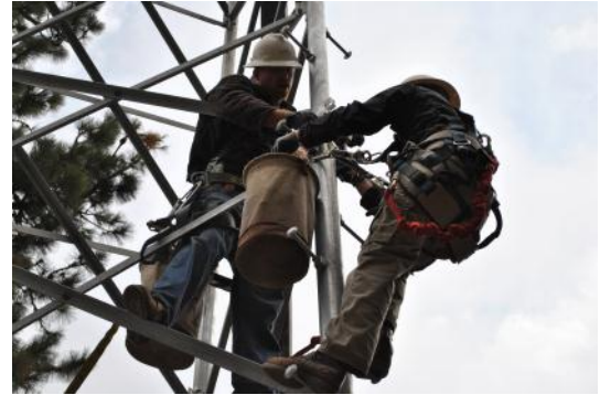
Construction workers bolt together two sections of a wireless tower.
