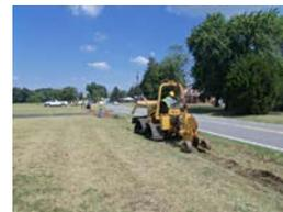
MBC using a vibrating plow to lay a fiber-optic network in southern Virginia.
