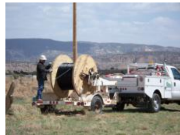
NTUA prepares to install new fiber in New Mexico.
