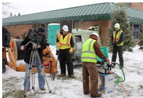
Merit Network crews begin to feed fiber into the conduit.
