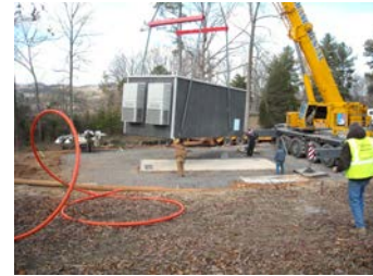
Deltacom crew installs a pre-fabricated building that will house fiber.
