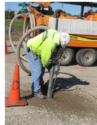
South Dakota Network crews have installed 72 miles of new fiber.
