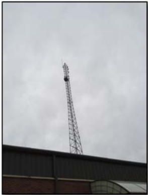
Transmit Tower at Gibson Electric
