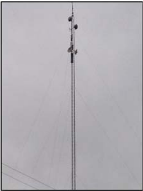
Fire Department Transmit Site
