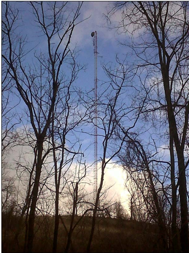
Exhibit B: Cable Head-End Location
